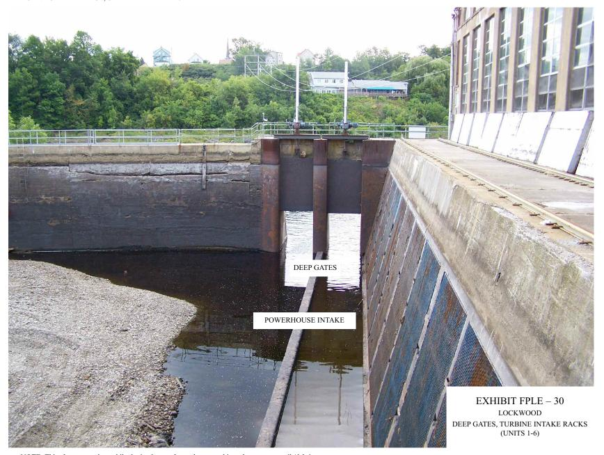
NOTE: This photo was taken while the intake canal was de-watered in order to remove silt/debris.
